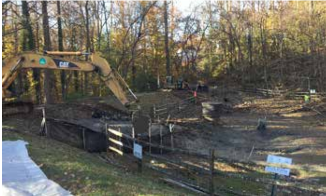
The poorly developed drainage area on Rannock has been removed of sludge allowing for good drainage.
